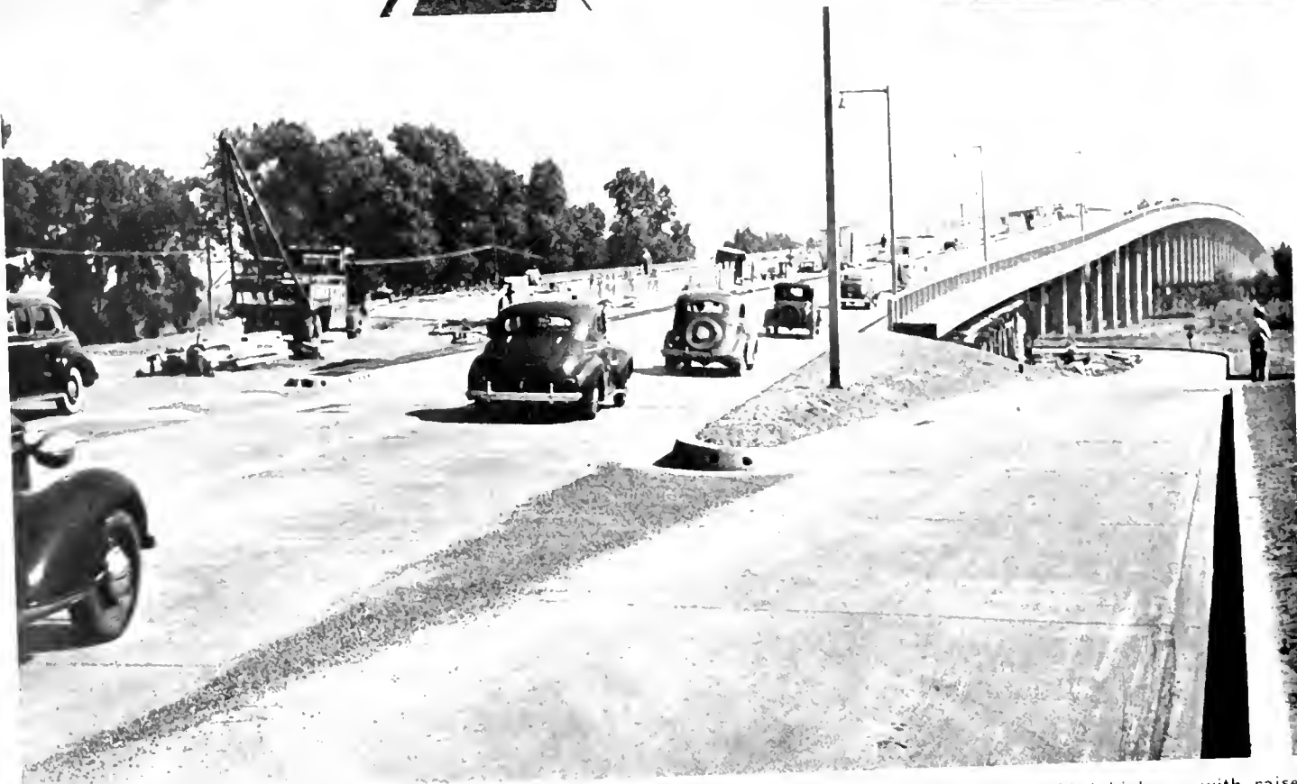
At top—Full width view of completed roadway of North Sacramento viaduct showing four-lane divided highway with raised curbed median strip, four feet wide. Each traffic lane is 25 feet wide. Bottom—View of east bound traffic using structure immediately after dedication. (See story on pages 3 and 16.)
